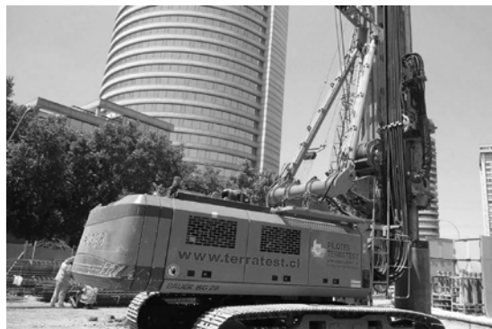
Figure 3. Bored cased piles being executed
